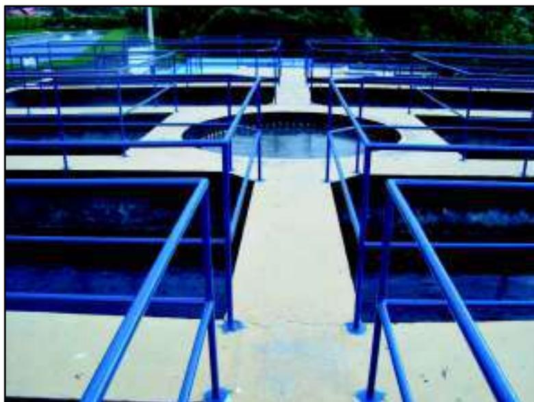
**Figura 7.81 - Reator UASB**
